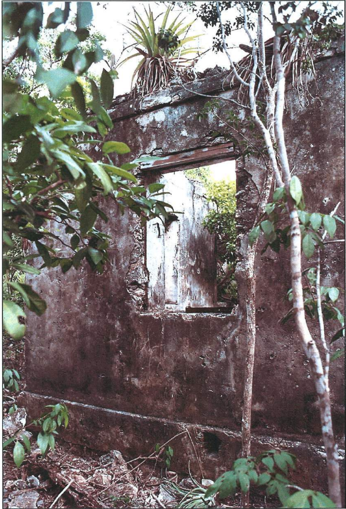
Plate I. 8: Alexandria, Structure in vicinity Plot Nos. 14 and 15. West facade.
